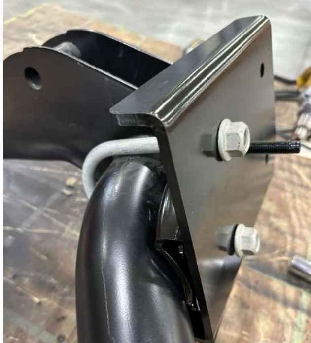
Photo 18: U-Bolt loose install
