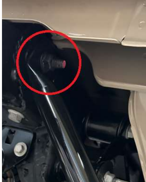
Photo 24: Pencil brace installation
