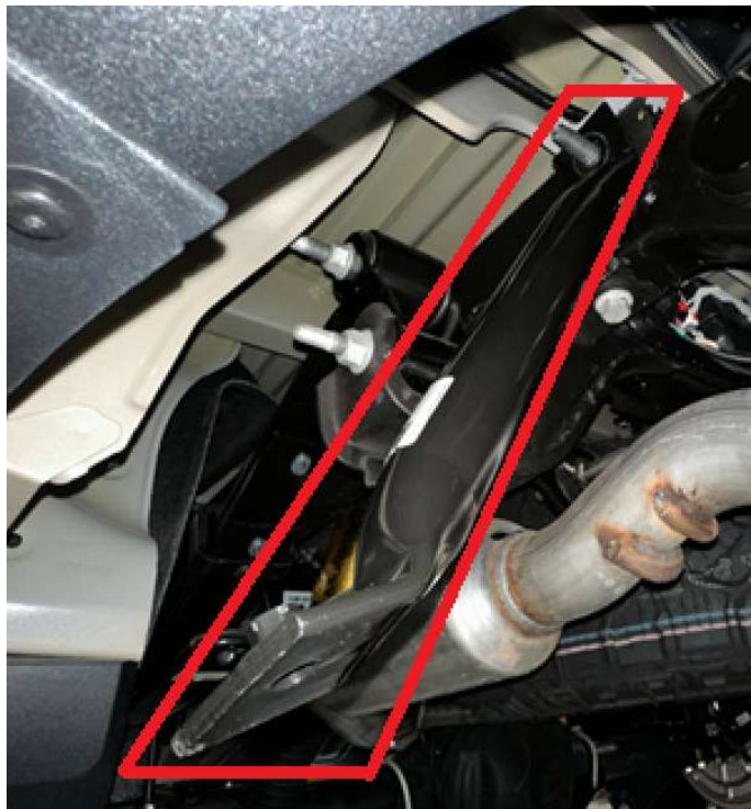
Photo 21: Pencil brace installation
